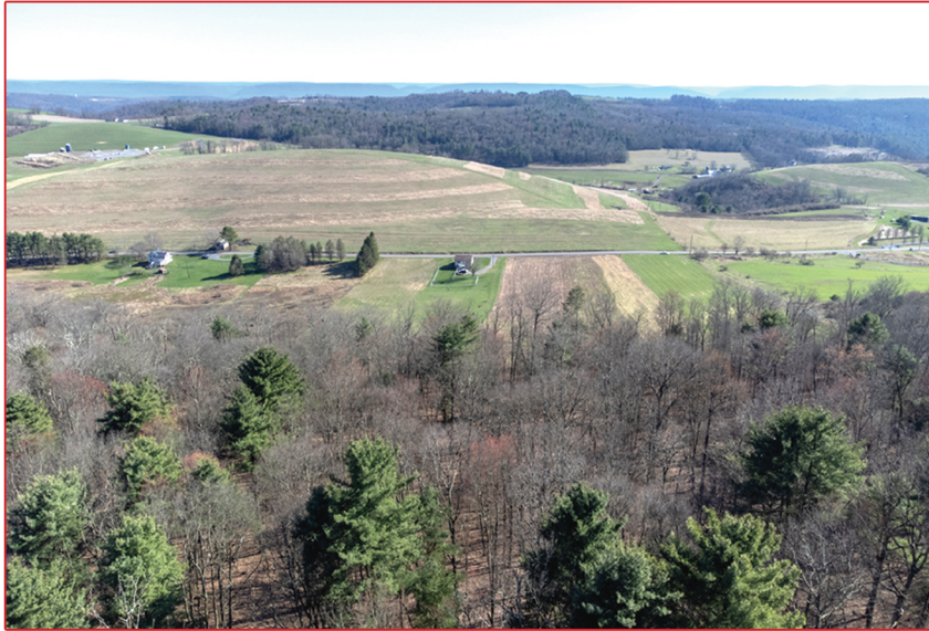
WEST ROUTE 973 HIGHWAY, COGAN STATION
